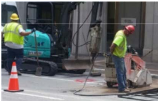
Worker using a walk-behind saw with an integrated water delivery system to cut asphalt roadway.
