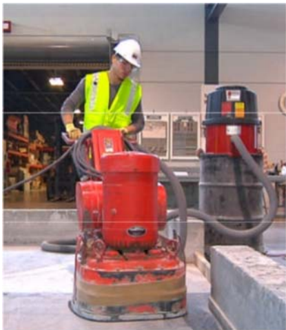
Worker milling granite floor indoors with milling machine and vacuum dust collection system (background).
