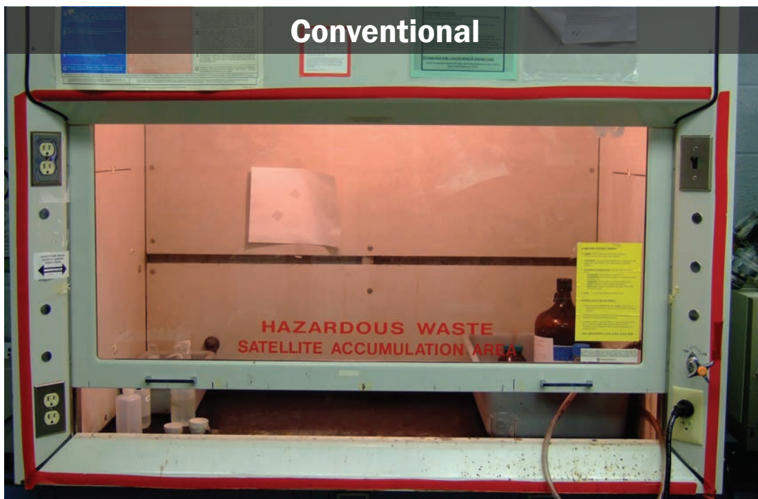
Figure 10. Conventional (constant-flow) laboratory chemical hood.
